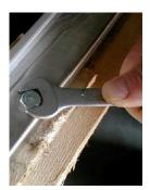
Unscrew the unit's frame from the wooden base.
