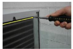
On the air cooled units, loosen the three screws enough to fit the air baffle plate into place.
